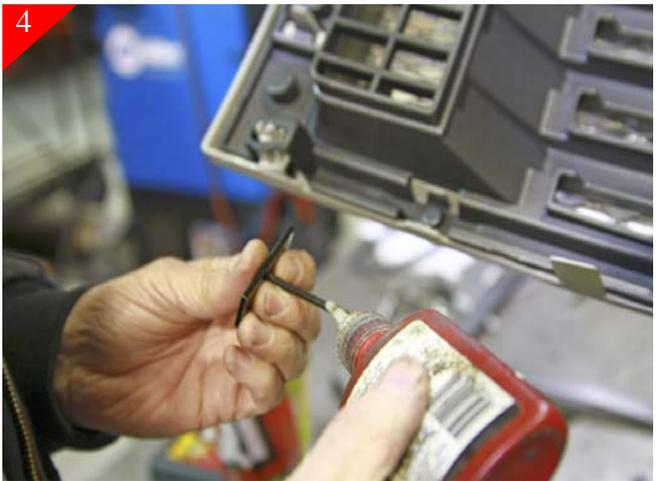
With brackets attached place stock shell face down on top of the mesh and the trim ring. Locate the 6 rectangle tabs and place the 10-24 x 1 1/2 bolts thru the center hole in tabs. Next place a drop of blue or red loctite on threads of the bolts.
