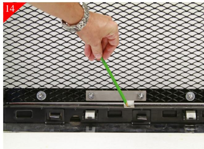
With bolts removed using a scribe mark hole locations. Next you will need to mark the drill locations for the brackets on backside of grill. Turn grill over and using a scribe mark the hole locations for the brackets as shown.
