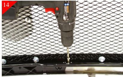
With all hole locations marked remove the mesh grille from opening. Using a 1/4" drill bit, drill the marked locations.
