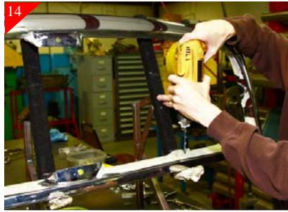
Next loosen brackets so that you can remove the mesh grille from opening. Using a 3/8" drill bit drill all marked locations.
