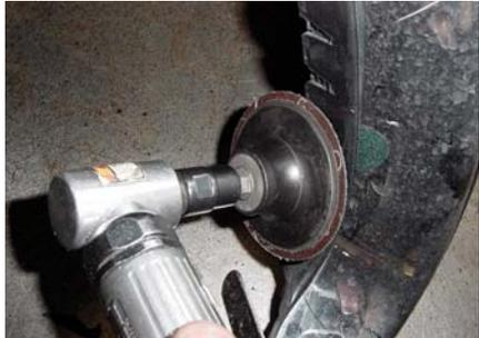
**STEP 6** Grind or Sand any raised areas flush with the black area.
