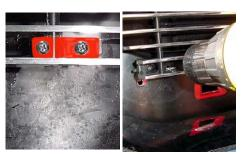
**STEP 9** Locate tab as shown and drill a 3/32" hole for each tab and attach using #8screws provided.
