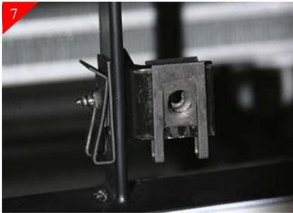
Now attach the brackets to the vertical supports in the just drilled locations. Using the supplied U-clips and #8 x 5/8" phillips head screw as shown above.
