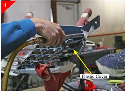
Using masking tape, tape the chrome portion of stock shell to protect during installation of billet grille. Lay grille shell face down. Now locate the plastic covers that are on the outer edge of the passenger and drivers side of the shell as shown above. Using a grinder remove the plastic weld tabs holding them in place and remove covers.
