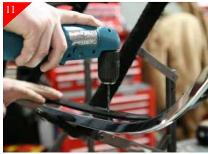
Using a 3/16" drill bit drill all the just marked areas.
