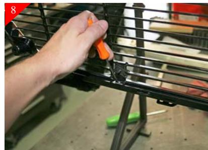
With the brackets held in place against the black plastic, using a scribe mark the hole locations in the brackets as shown above.
