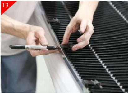
Mark the center location of the hole in all (4) just placed brackets where it meet the stock shell as shown above.
