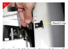
Locate supplied bottom brackets and place u-clip on bracket as shown above. Attach bottom brackets by placing brackets in the (2) inner most slot openings as shown then place a supplied U-clip on the under side of grille opening. Then using the supplied #8 x 5/8" screw tighten brackets.
