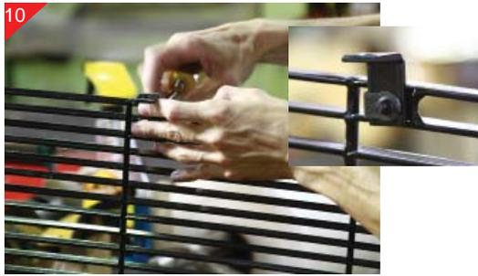
Next attach the top center bracket to billet grille using 10-24 clip and 10-24 x 5/8" bolt as shown.
