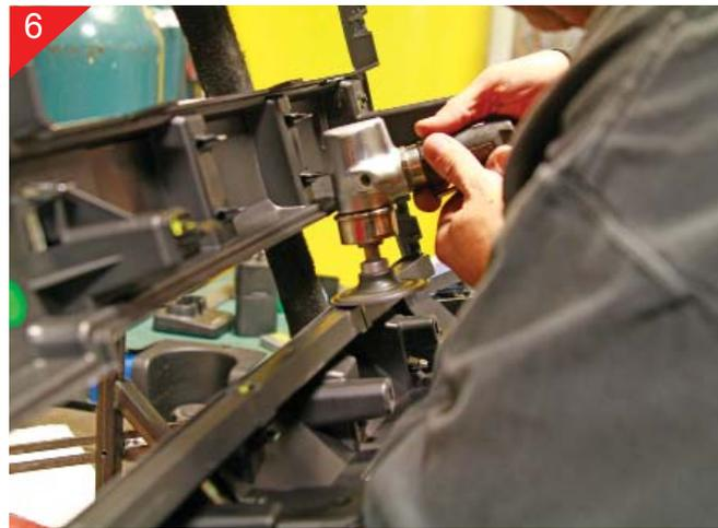
You will need to sand all cut areas smooth with surface of grille shell using a air sander or sanding block.
